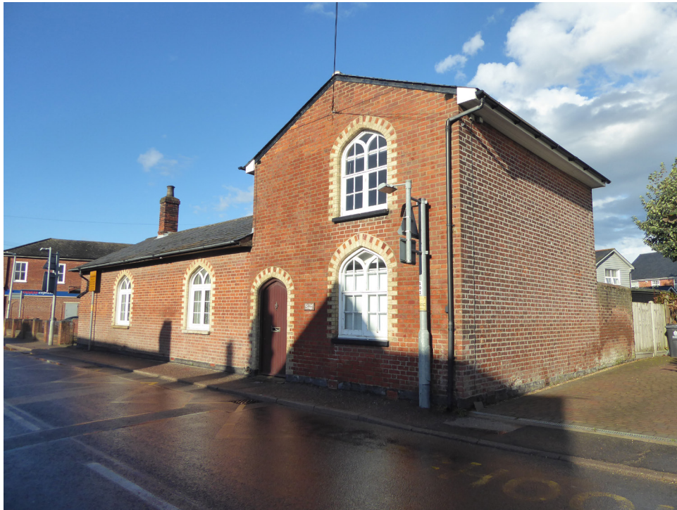
Figure 25 Photograph of Old Hall Cottage
